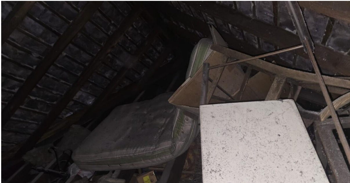
Plate 7: Image of the stored items within the roof void of B1 .
