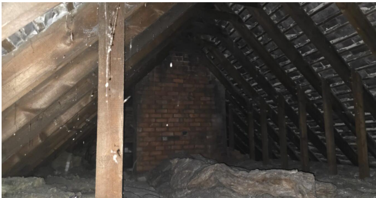
Plate 5: Image showing the internal roof space within B1 including cobwebs.
