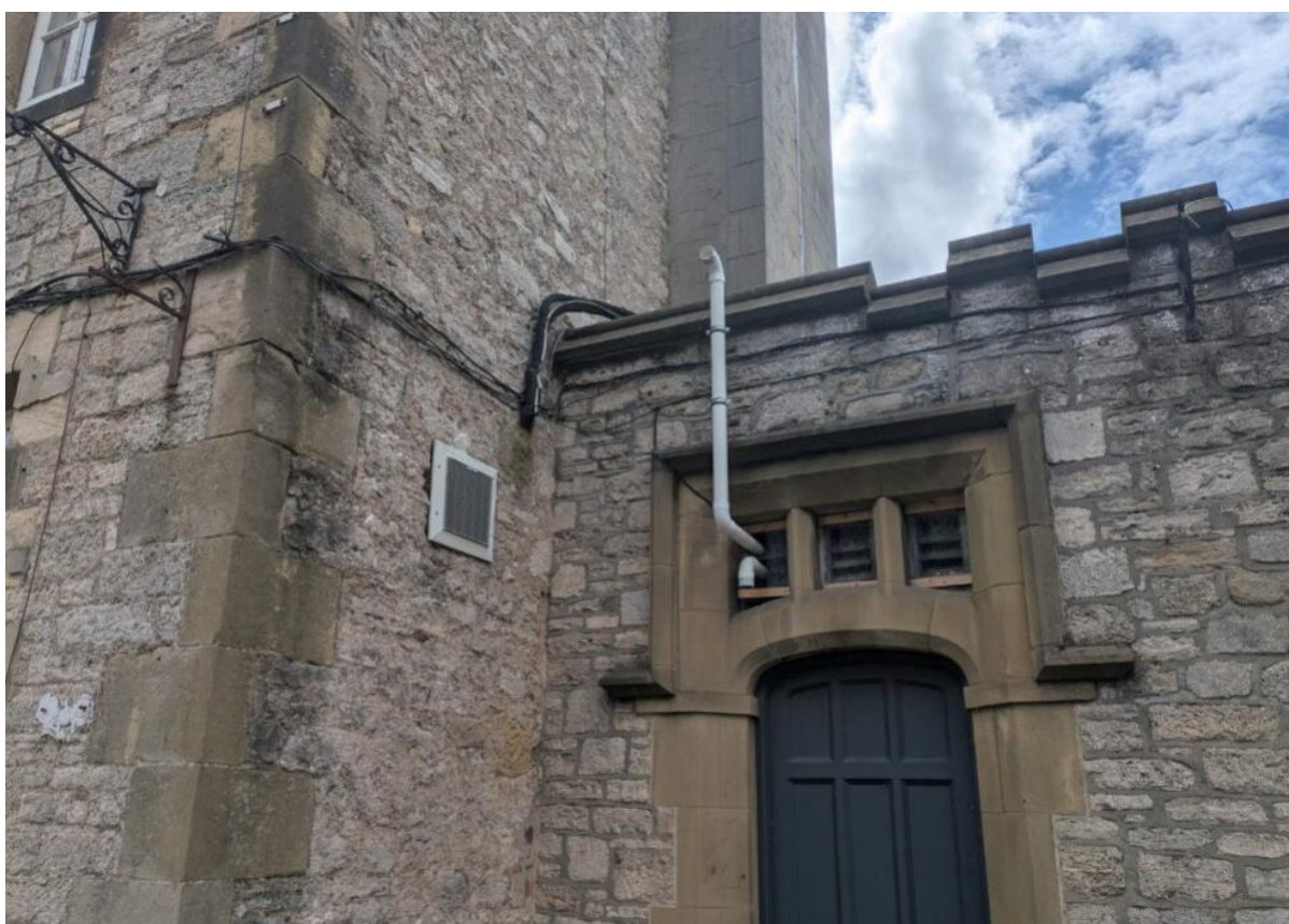
Plate 4: Image showing the vent present on the southern elevation of B1 .
